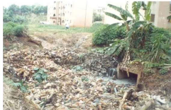
Lack of sanitation facilities in urban settlements
